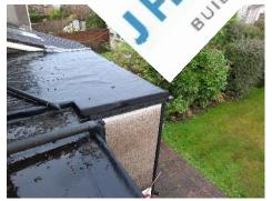
4. The leadwork stops short and there is a gap existing boundary wall / adjoining property's pitched ror the entry of insects or rodents into the void  $\varepsilon$ maintaining an air gap.
