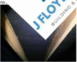
7. The existing roof insulation, while in good condition it do approximately 300mm thick. If additional insulation w<sup>-</sup> costs and improve the level comfortability.
